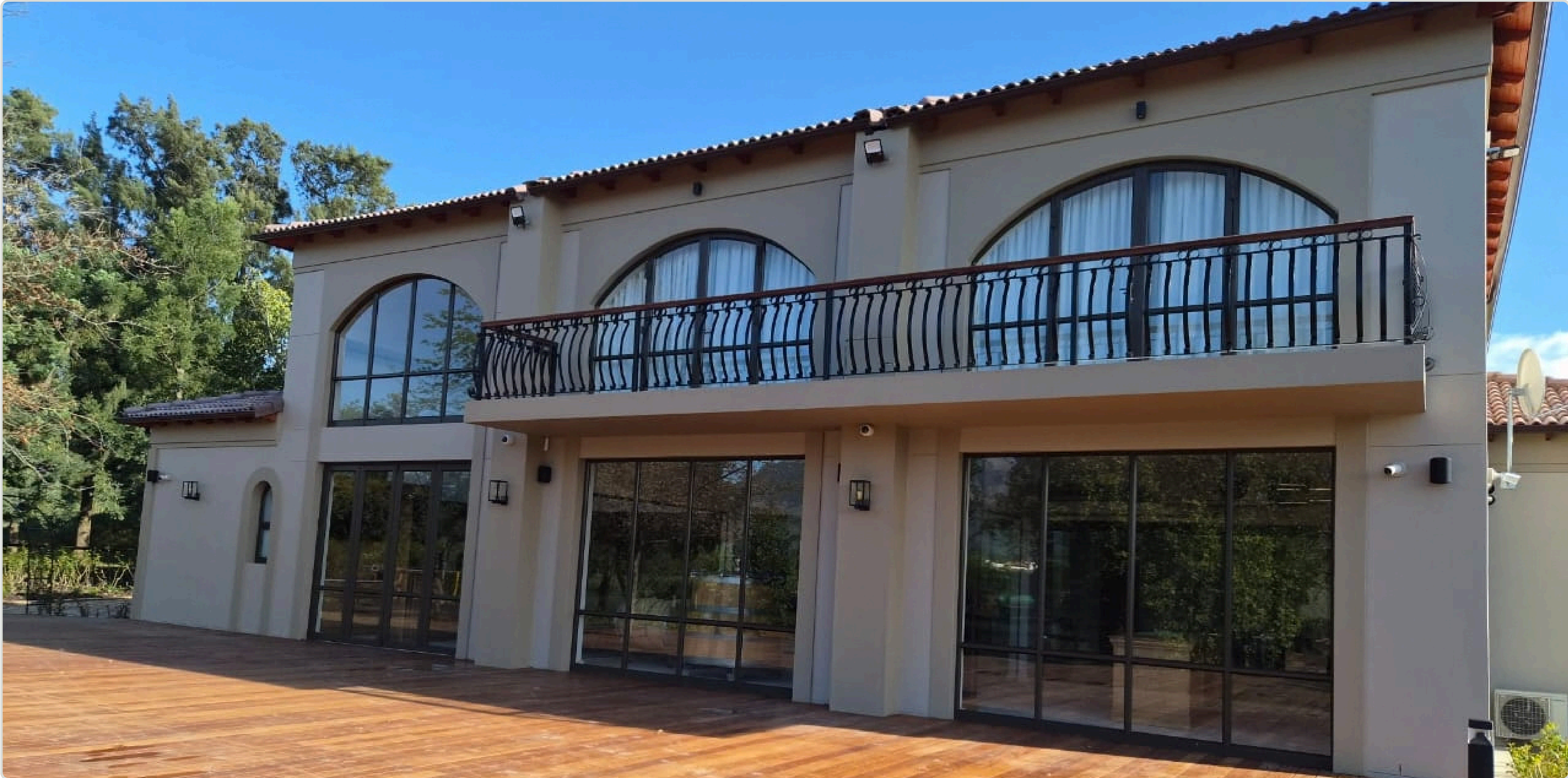
Santé Cellar | Paarl | Custom aluminium window installation & glazing
