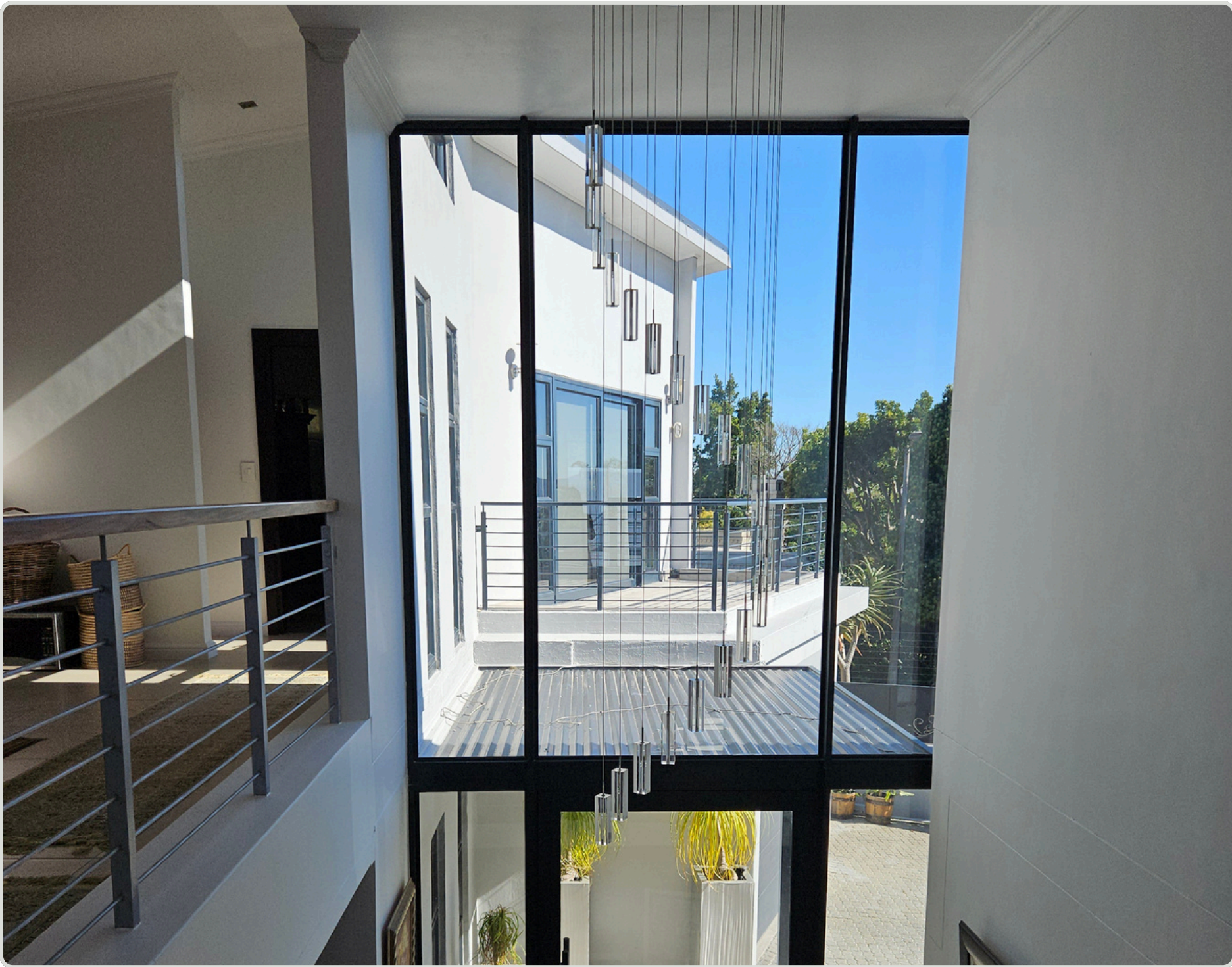
Residential | Paarl | Custom glazing and fixed aluminium window solutions
