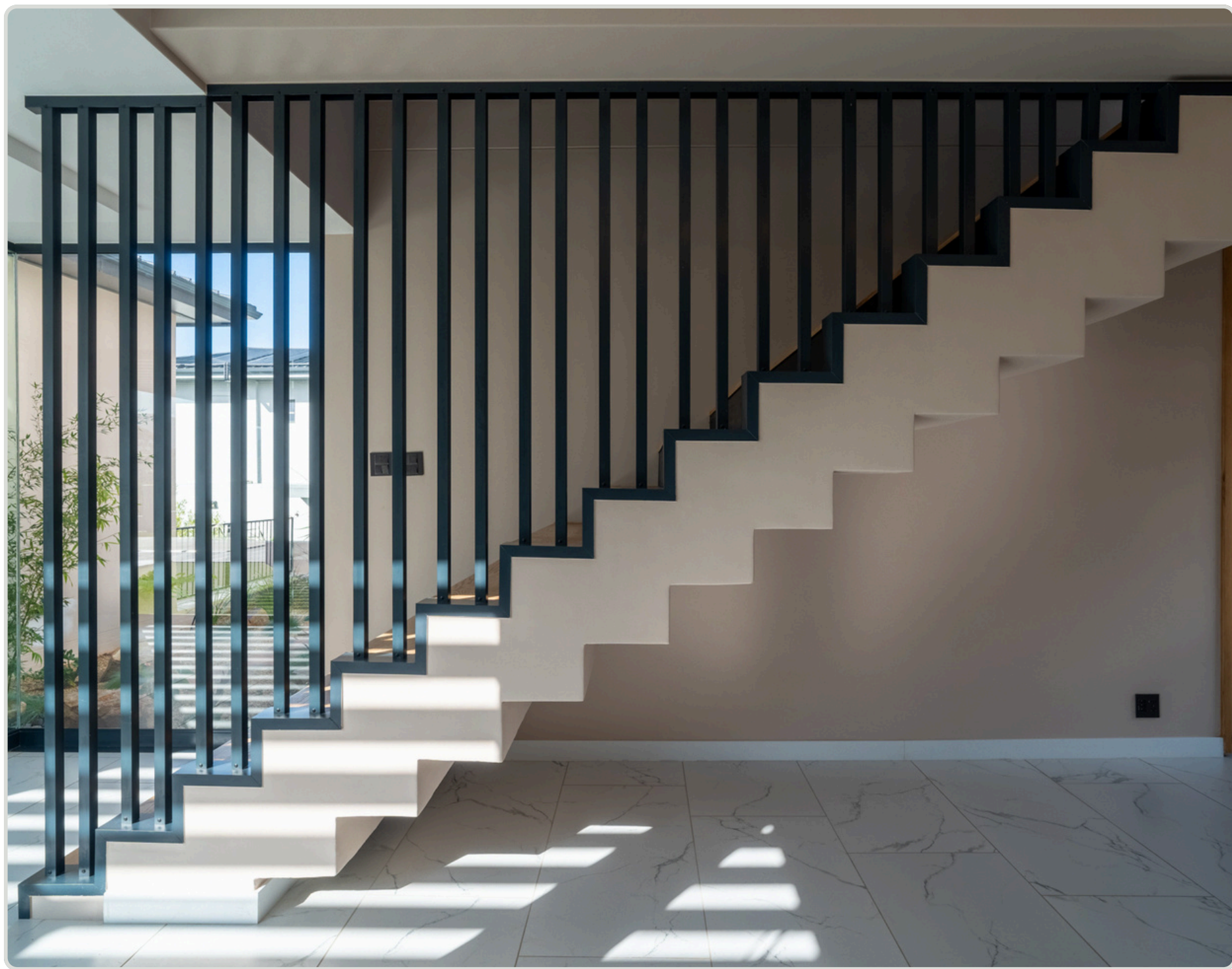
Architectural | Screening | Vertical aluminium screening integrated into the building to define space and provide separation.
