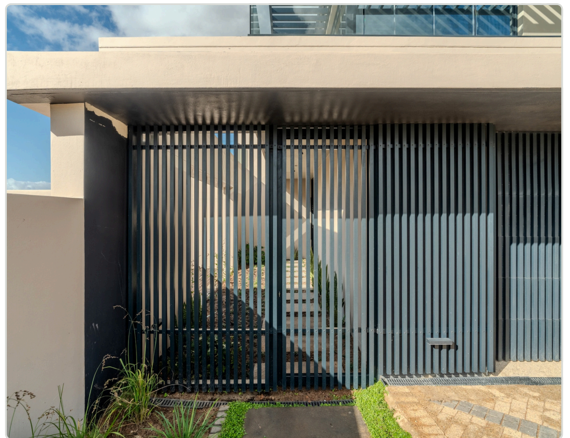
External aluminium screening | A full-height aluminium screen designed around the entrance, adding privacy and definition to the façade.
