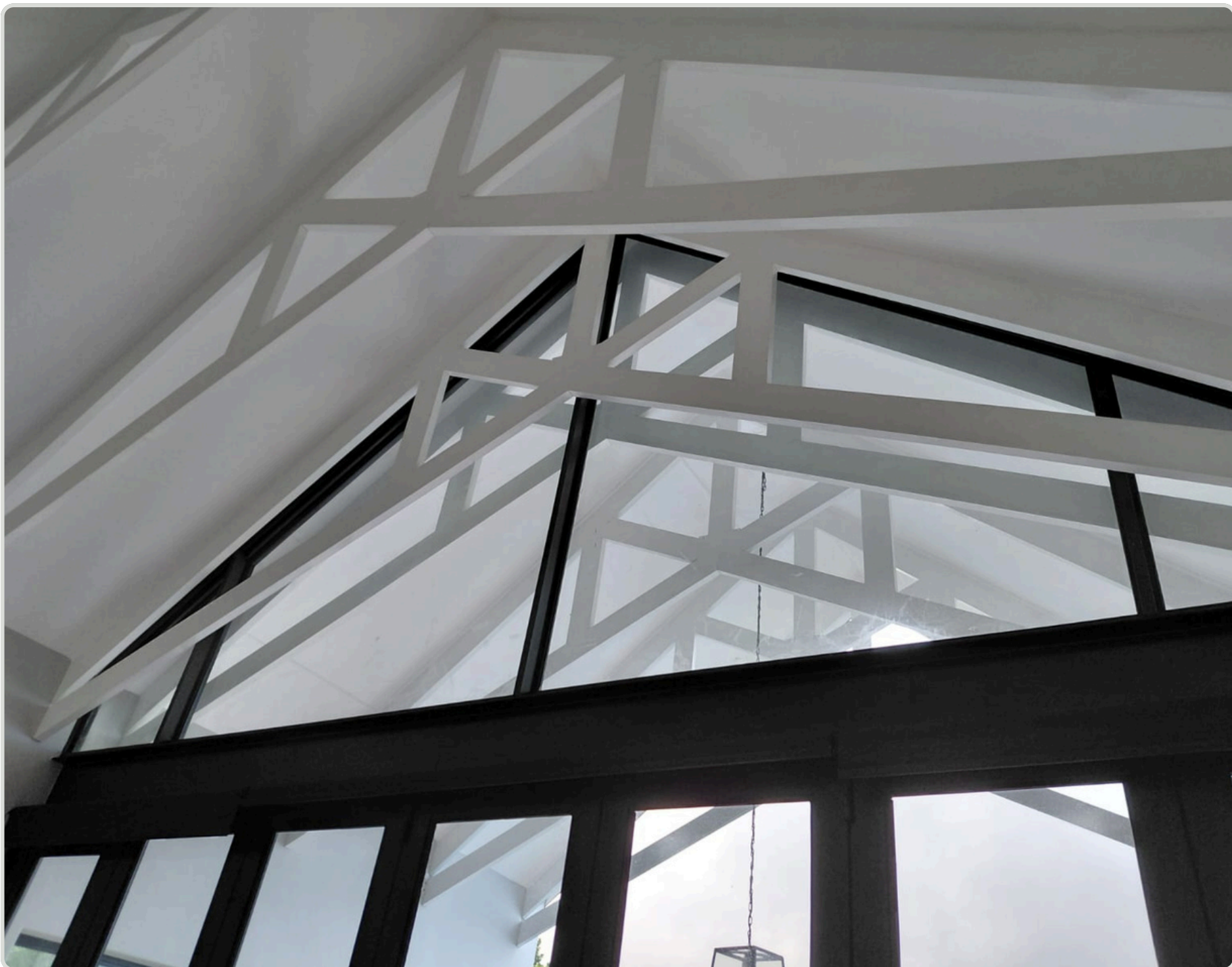
Architectural | Feature Glazing | Custom glass fitted within the structure and geometry of the building
