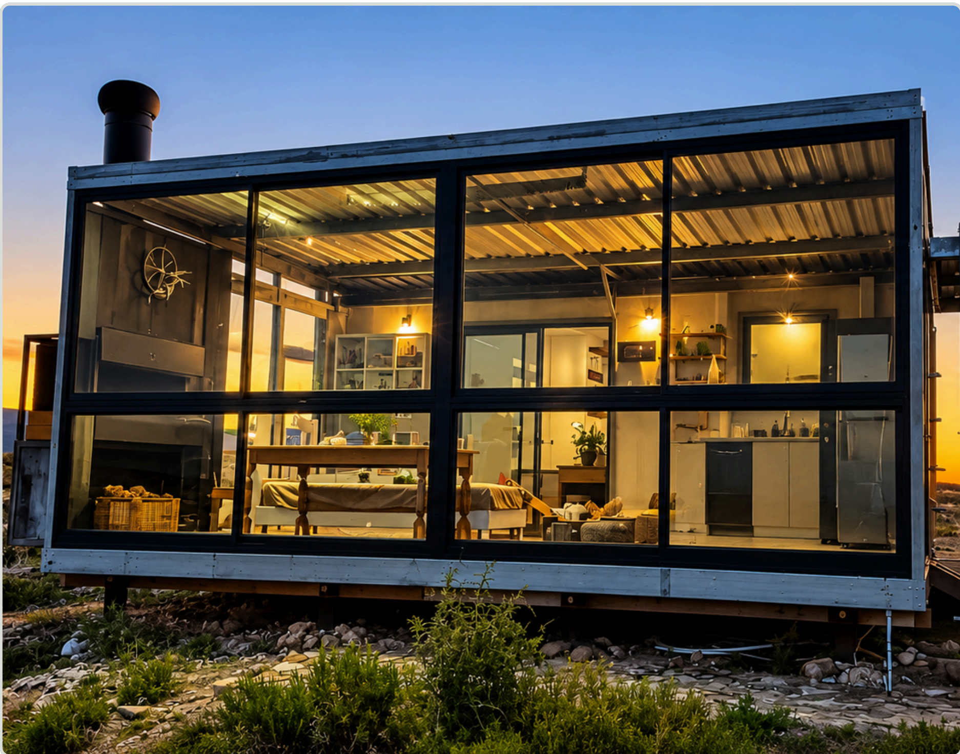
Residential | Custom Glazing | Glass solutions integrated into a contemporary residential project
